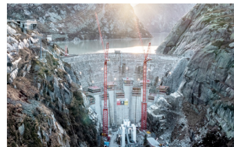
Spittallamm Dam, © David Birri
