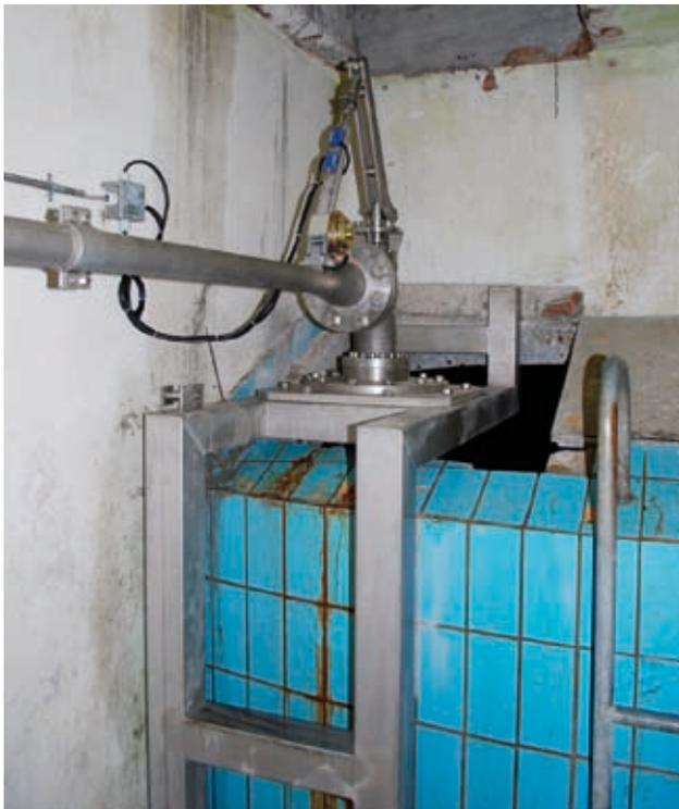
Photo 26. A Carnot bypass equipped with an adjustable nozzle set against the reservoir wall
