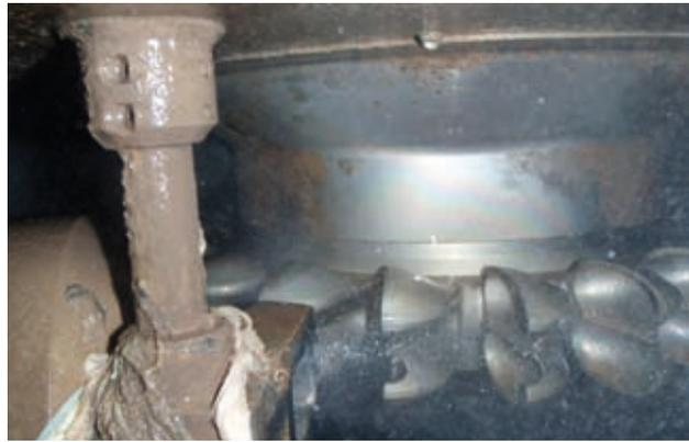
Photo 23. A deflector in the raw wastewater of Profray SHP plant (case study n° 11)
