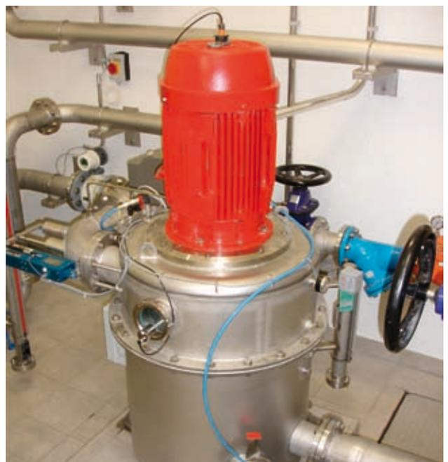
Photo 19. Counter pressure Pelton turbine (Fällanden SHP plant, Switzerland, set in a drinking water network,  $\Delta Z = 140$  m,  $Q_n = 16$  l/s, 17 kW, 2008)
