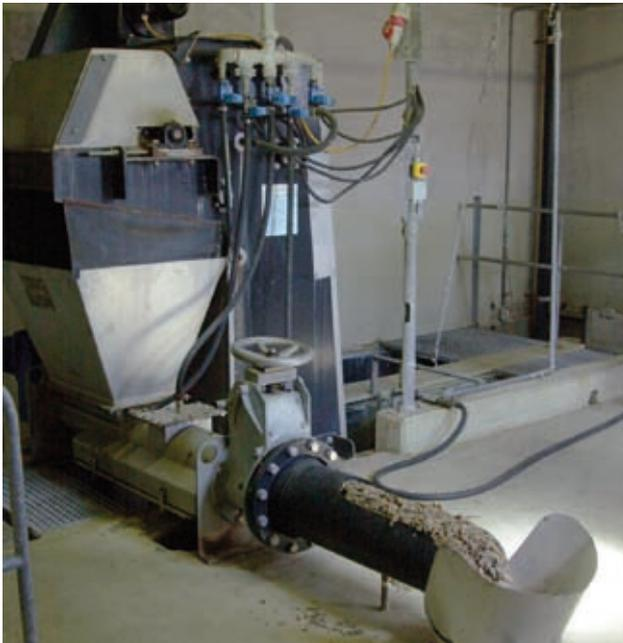
Photo 9. Screening system for wastewater at the forebay (Profray power plant, Switzerland, case study n°11)
