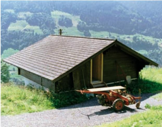
Photo 1. Trois Torrent power house, set in a drinking water network (Switzerland) ( $\Delta Z = 242$  m,  $Q_n = 35$  l/s, 70 kW, 1999)
