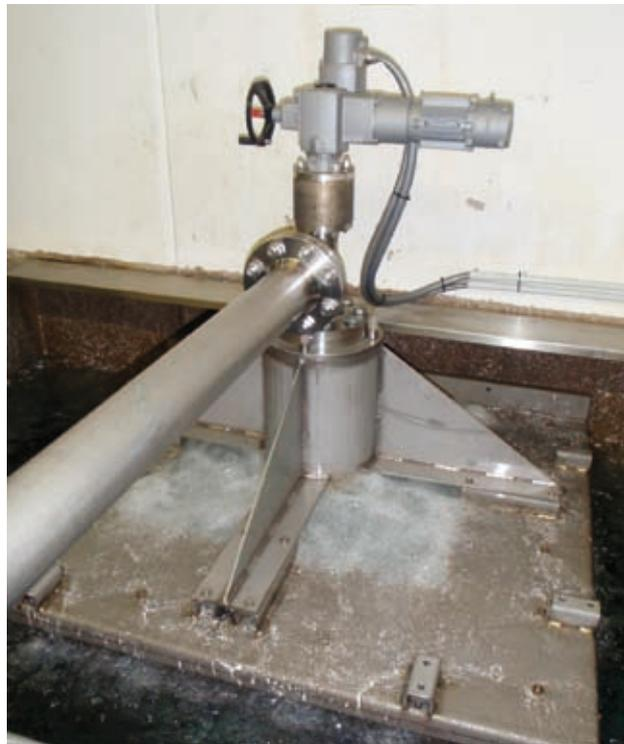
Photo 27. The Carnot bypass in operation
