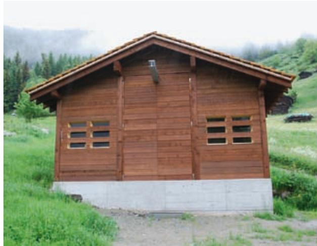
Photo 2. St Jean power house, set in a drinking water network (Switzerland) ( $\Delta Z = 373$  m,  $Q_n = 34$  l/s, 102 kW, 2009)
