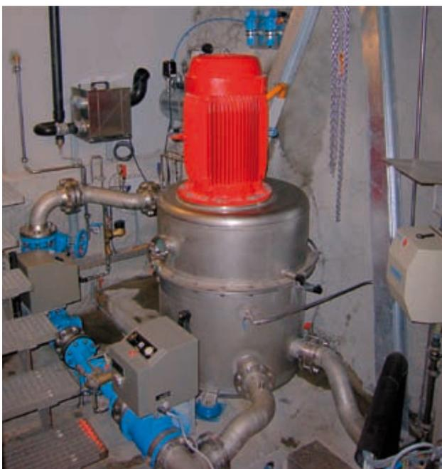
Photo 18. Counter pressure Pelton turbine (Mels SHP plant, Switzerland, set in a drinking water network,  $\Delta Z = 415$  m,  $Q_n = 13$  l/s, 41 kW, 2008)
