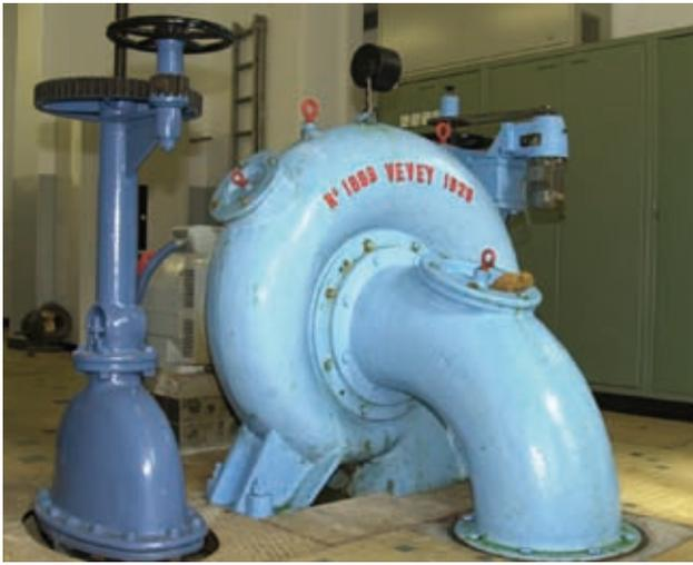
Photo 13. Francis turbine with a spiral casing set on the drinking water of Vallorbe (Switzerland)
