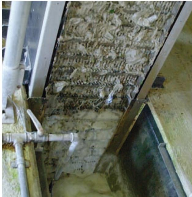
Photo 10. 6 mm grid for wastewater at the forebay (Profray power plant, Switzerland, case study n°11)
