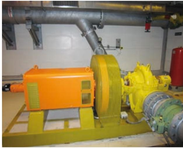
Photo 14. Reverse pump set on the treated wastewater of Nyon (Switzerland) (case study n°14)
