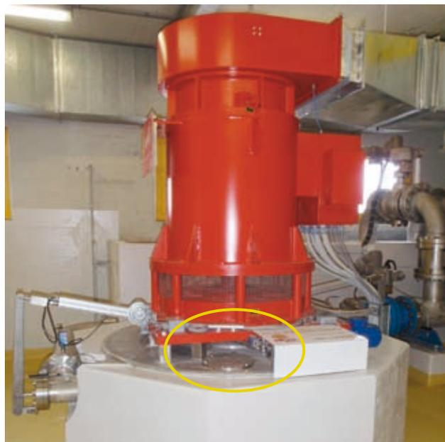
Photo 25. A hand hole with its cover, Profray SHP plant (case study n° 11)
