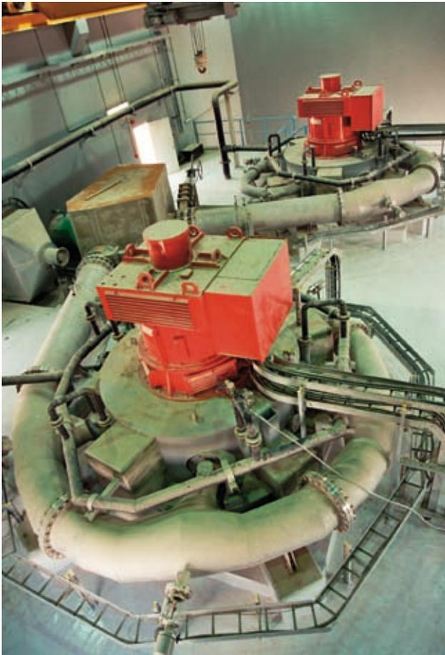
Photo 5. Two 5 nozzle Pelton turbines set on the raw wastewaters of Amman City, As Samra plants (Jordan)
